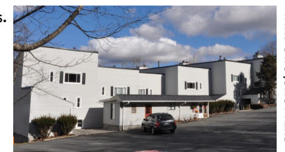
AFTER NEW! WINDOWS / SHUTTERS
